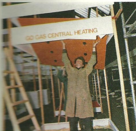
...the roof to one of the stands goes up...
