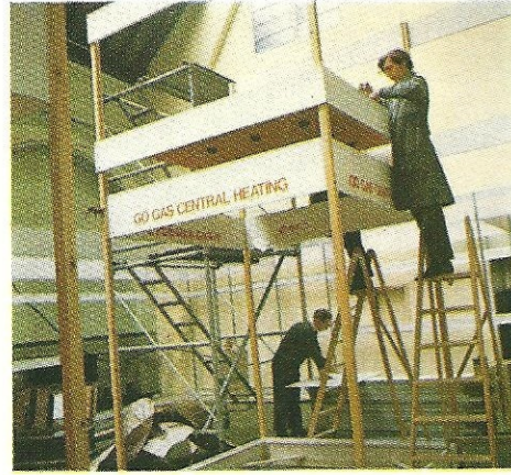
...one of the prefabricated units is erected...
